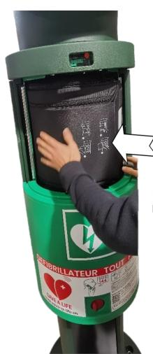
Position the cover against the bottom of the Aivia SOLO
