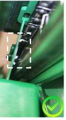
The runner is properly engaged. The door is properly fire2
